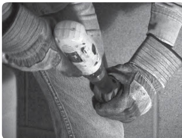
Solution: Using wire brush with power driver
