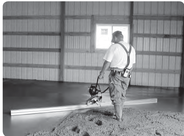
Solution: Motorized screeding
