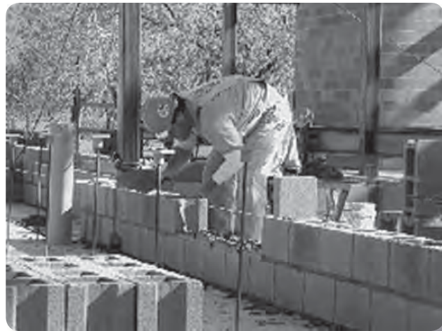
Problem: Laying standard concrete block
