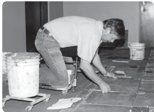
Solution: Laying tile with kneeling creeper
