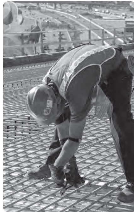
Problem: Tying rebar by hand
