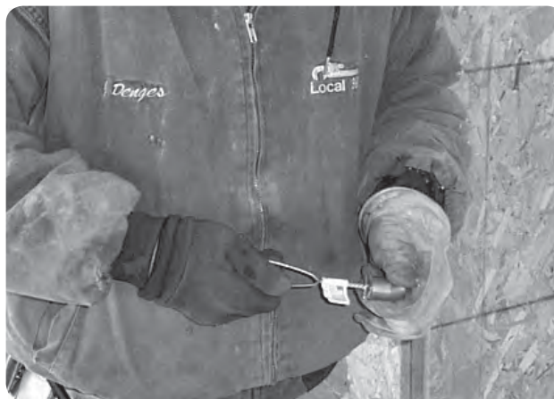
Problem: Brushing copper tube by hand
