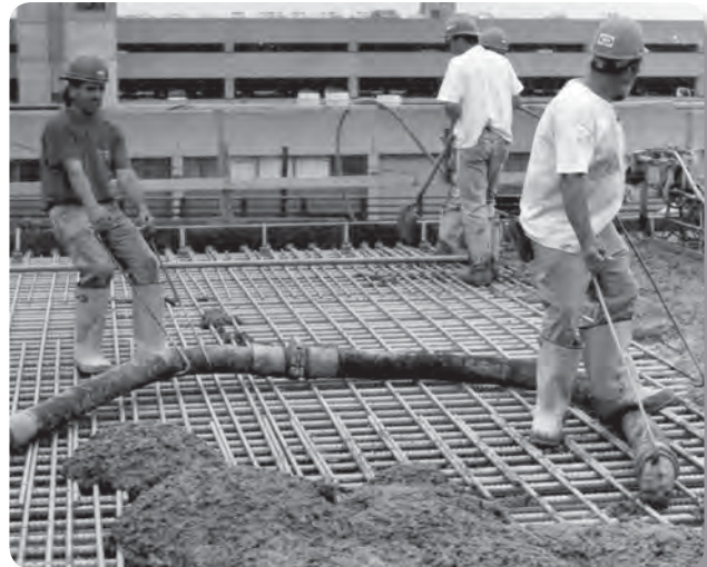
Problem: Pulling concrete hose without skid plate
