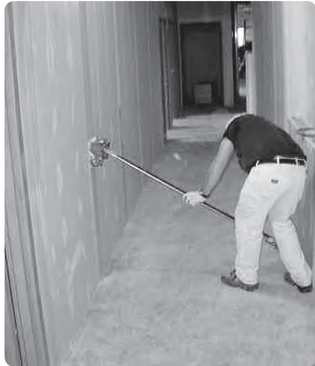
Problem: Hand drywall finishing with mudbox
